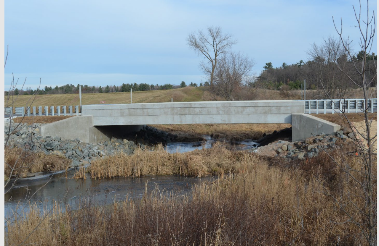
Example Bridge from a different project.
