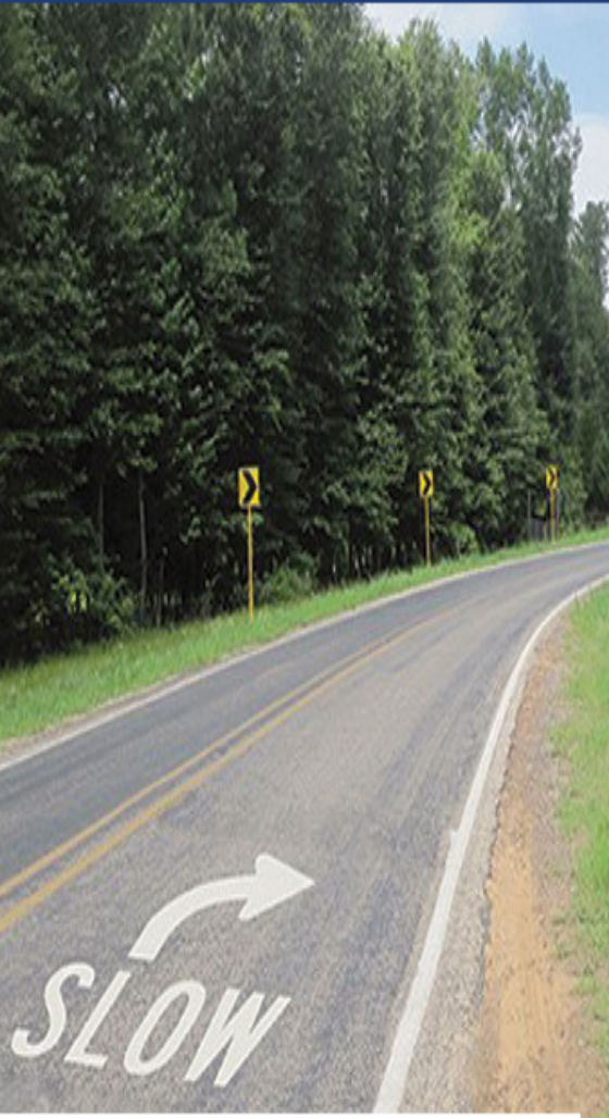
Figure 5. Curve delineation enhancements may include in-lane curve warning pavement markings and chevron signs with retroreflective strips on sign posts. Source: FHWA
