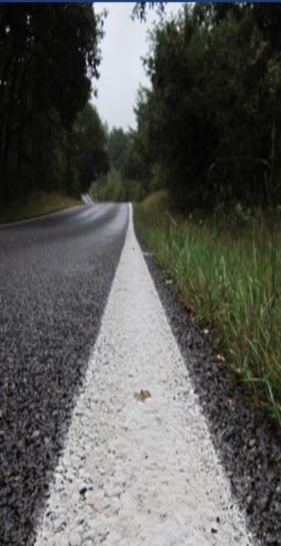
Figure 3. Wider edge lines enhance visibility of the travel lane. Source: Thurston County, WA
