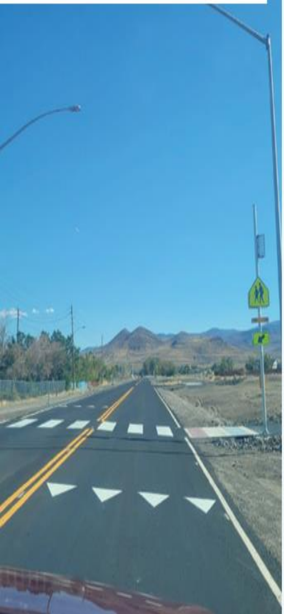
Figure 10. Crosswalk visibility enhancements include advance yield markings, high visibility crosswalk markings, lighting, and a rectangular rapid flashing beacon. Source: FHWA
