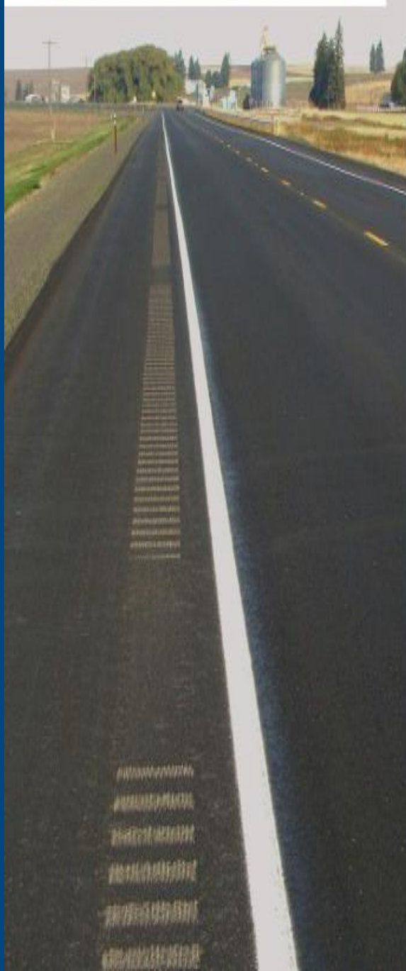
Figure 4. Shoulder rumble strips. Source: FHWA
