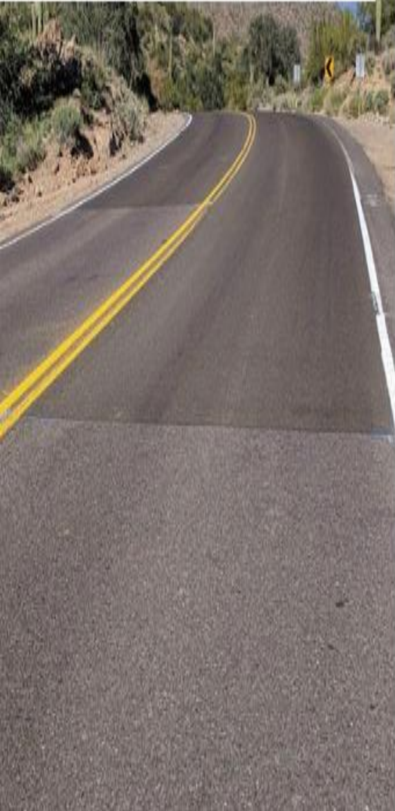
Figure 12. HFST applied at a horizontal curve. Source: Maricopa County, AZ
