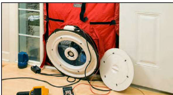
Blower door test being performed.
