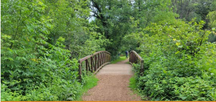
Bridge over creek
