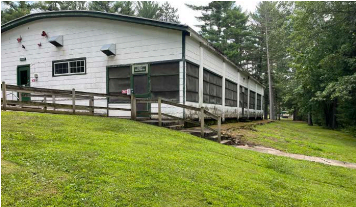
Existing building being considered for removal
