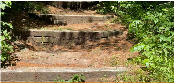
Existing stairs to beach
