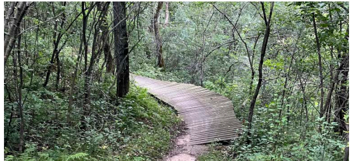
Path infrastructure for biking
