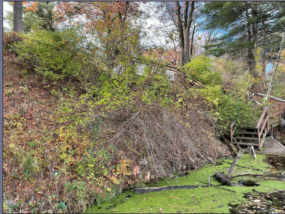
PHOTO TAKEN 11/3/2021 OF EXISTING SHORELINE CONDITION
