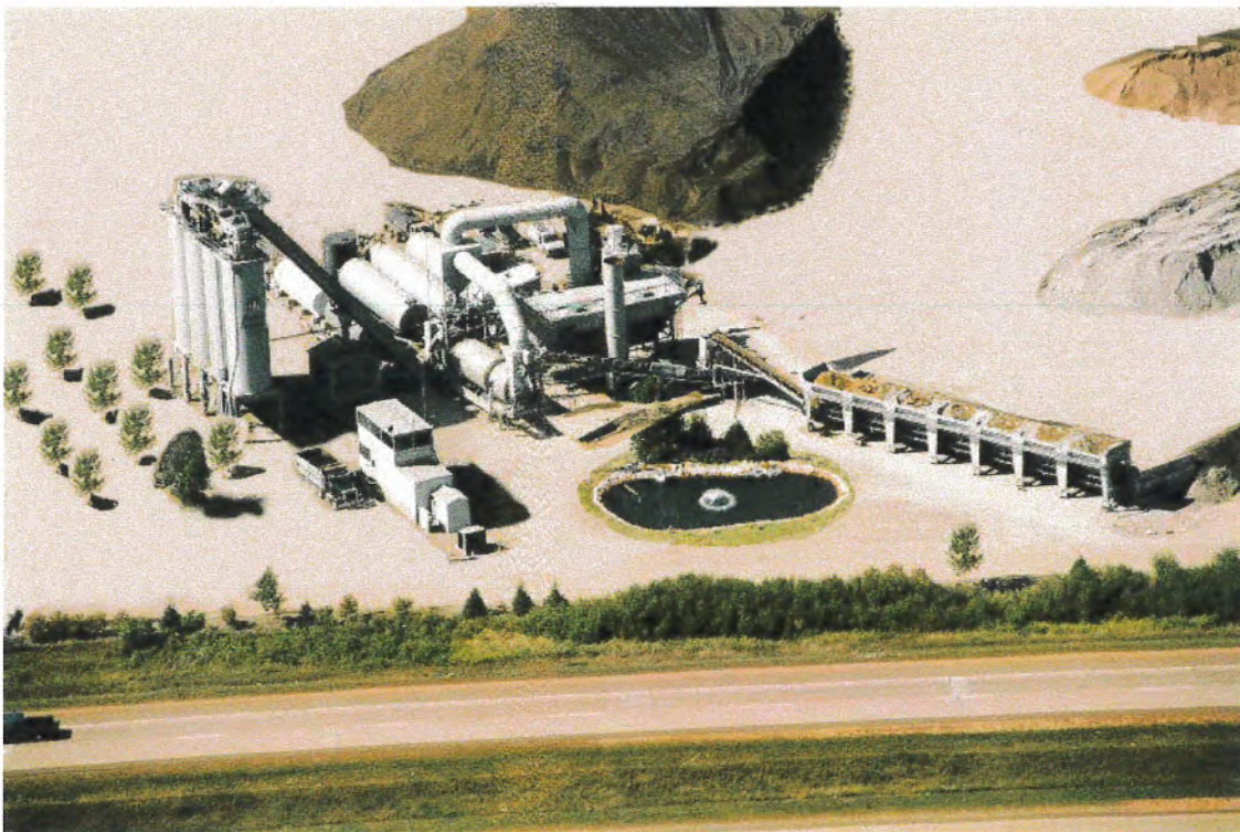
Photo 1, Typical HMA Plant Layout
