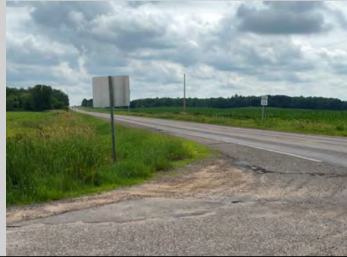
Looking east @ CTH SS & CTH GG (110 th Street)
